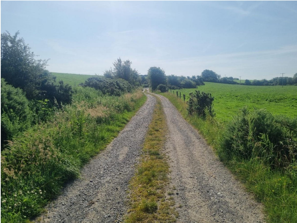
Photo 33 – Section of the local road L18062 subject to widening on the north (left) side (FW11)
