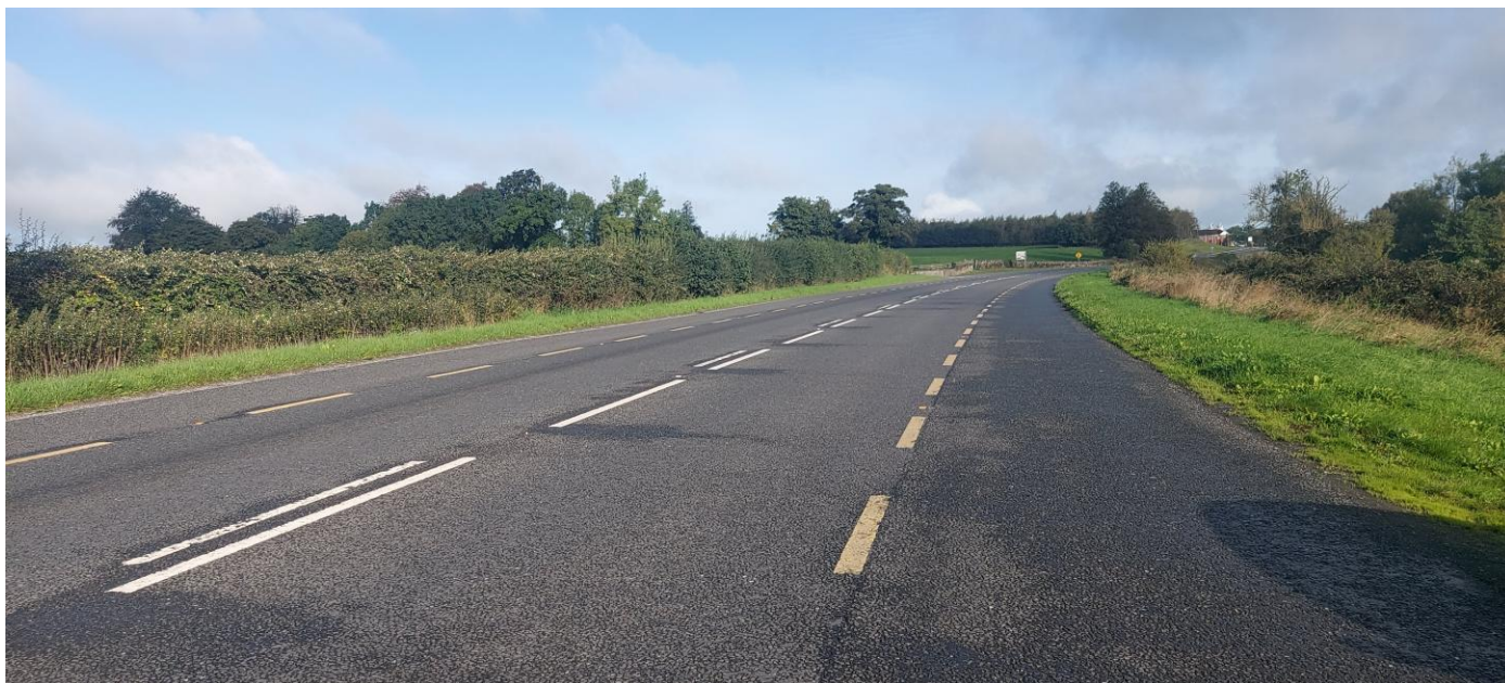
Photo 19 – Location of the Parksgrove-Moatpark UGC N77 national road horizontal directional drill
