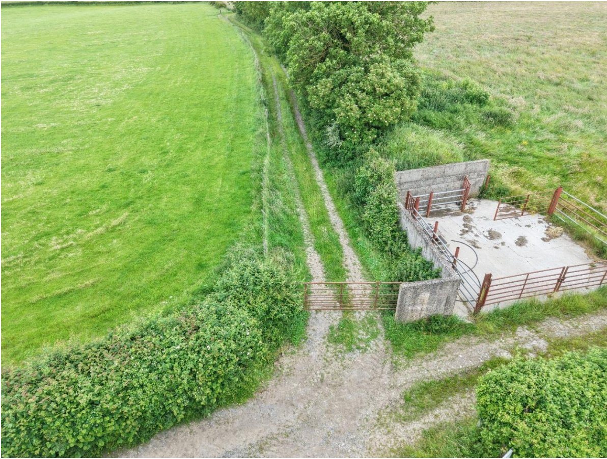
Photo 5 - Site Entrance 1 looking north and Location of Facilitating Works FW3 and FW4
