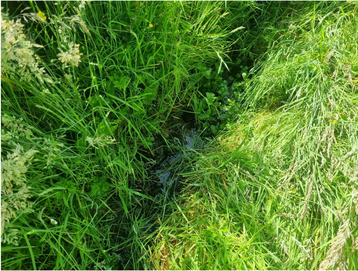
Photo 43 – Drainage channel D02
