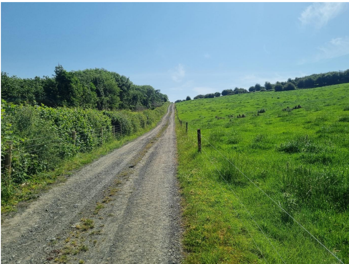
Photo 12 – Access road to T3
