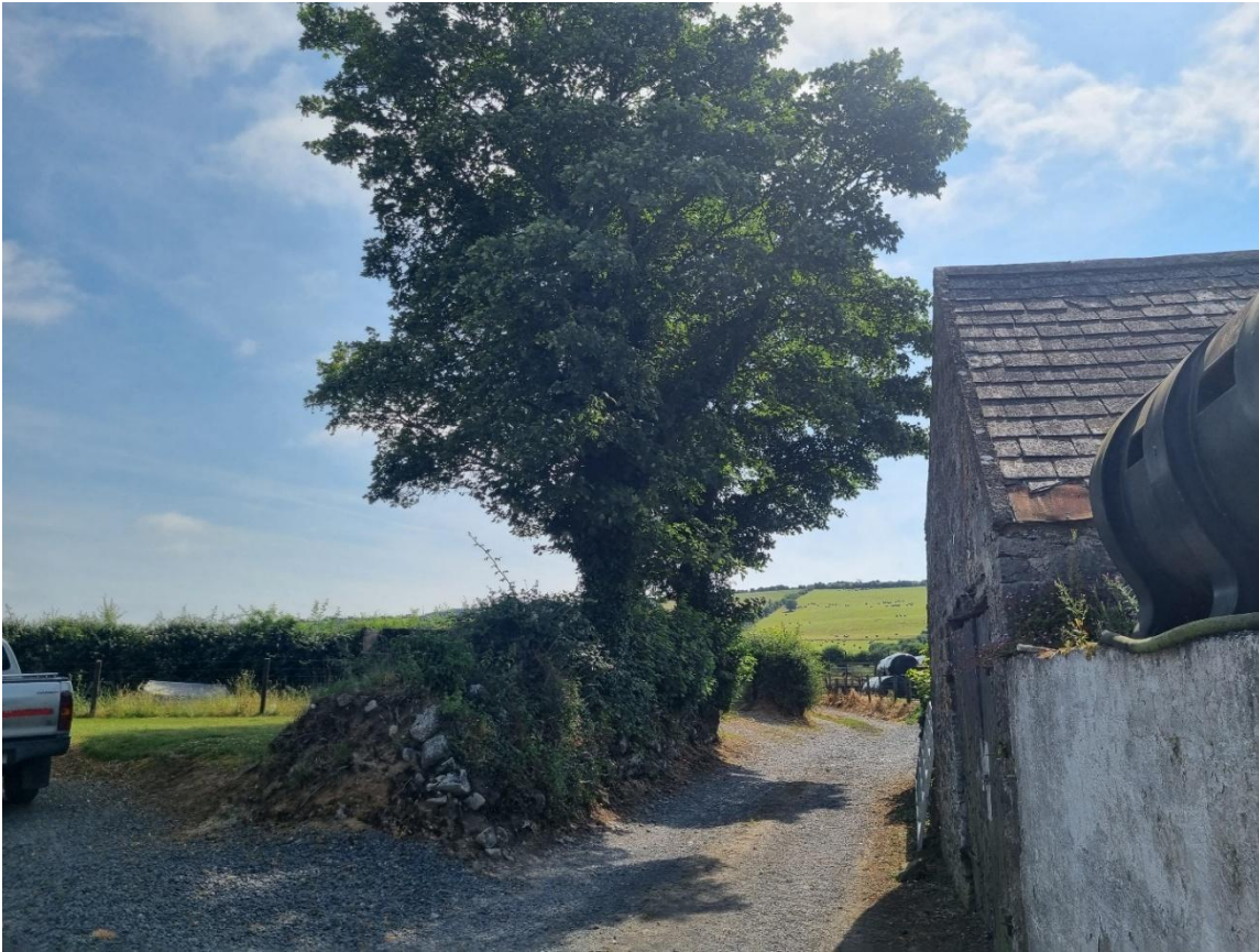
Photo 3 – Section of the local road L58141 subject to widening on the north (left) side (FW2)
