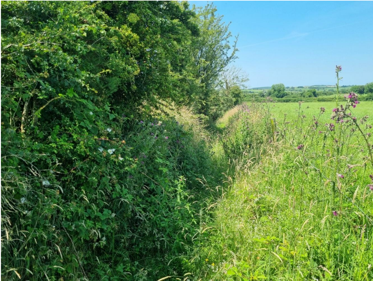
Photo 35 – Drainage channel D01
