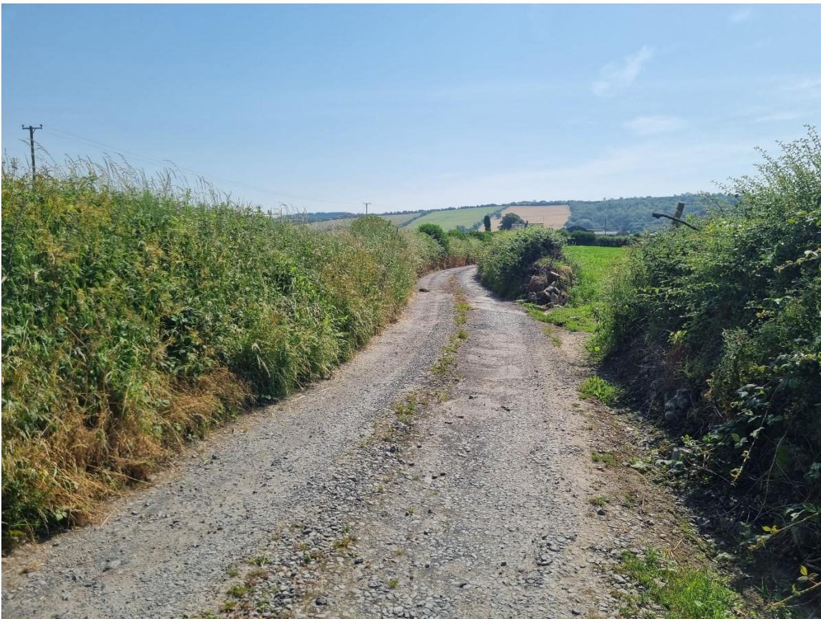
Photo 2 – Section of the local road L58141 subject to widening on the south (right) side (FW2)
