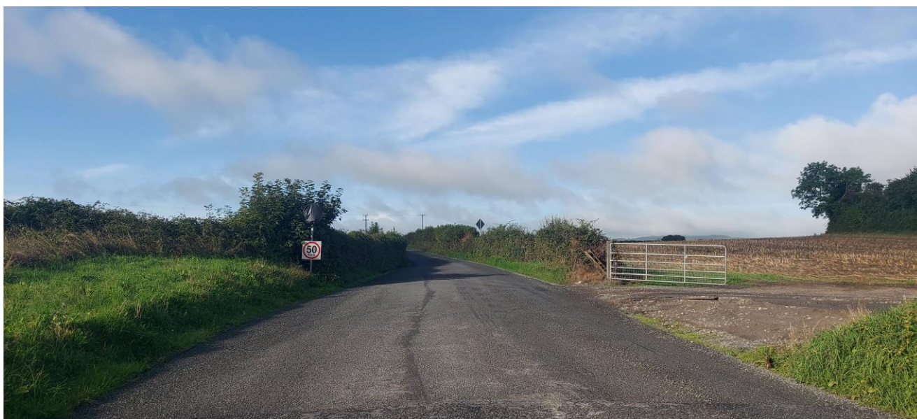
Photo 16 – Location of the Ballyring-Parksgrove UGC L1807 local road crossing
