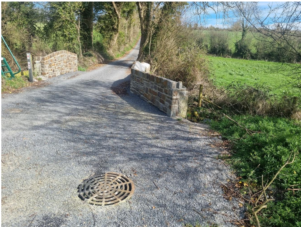
Photo 4 – Location of the Ballylehaun-Ballyring UGC watercourse crossing (W2) in the L5820 local road
