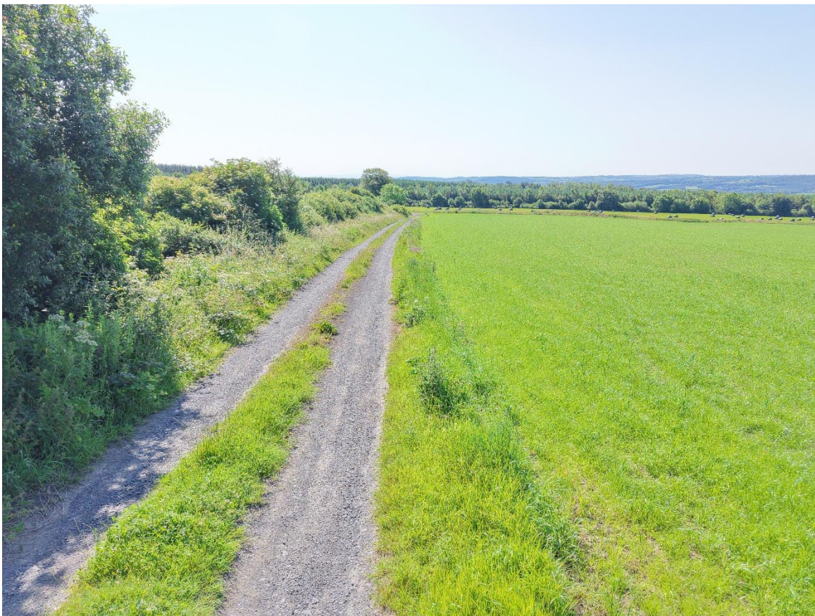
Photo 46 – Access road to T12
