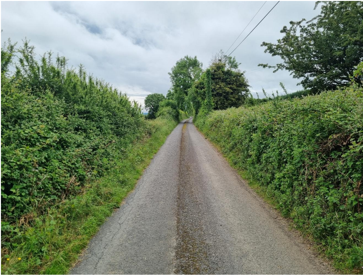
Photo 1 – Location of the Ballylehaun-Ballyring Underground Cabling (UGC) in the L5818 local road
