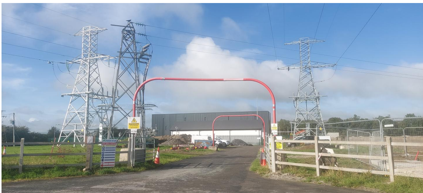
Photo 24 – Location of the Existing Eirgrid Ballyragget Substation in Moatpark townland
